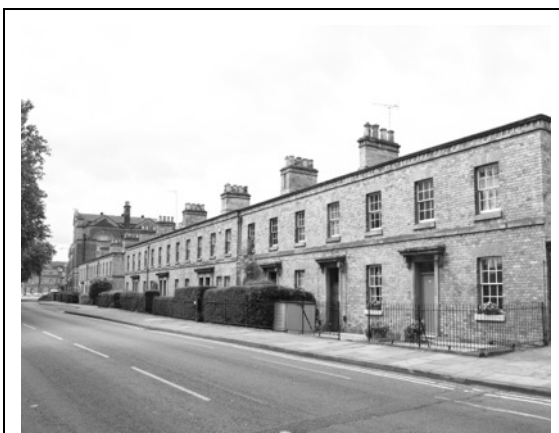
The once derelict and now restored cottages on Railway Terrace.
